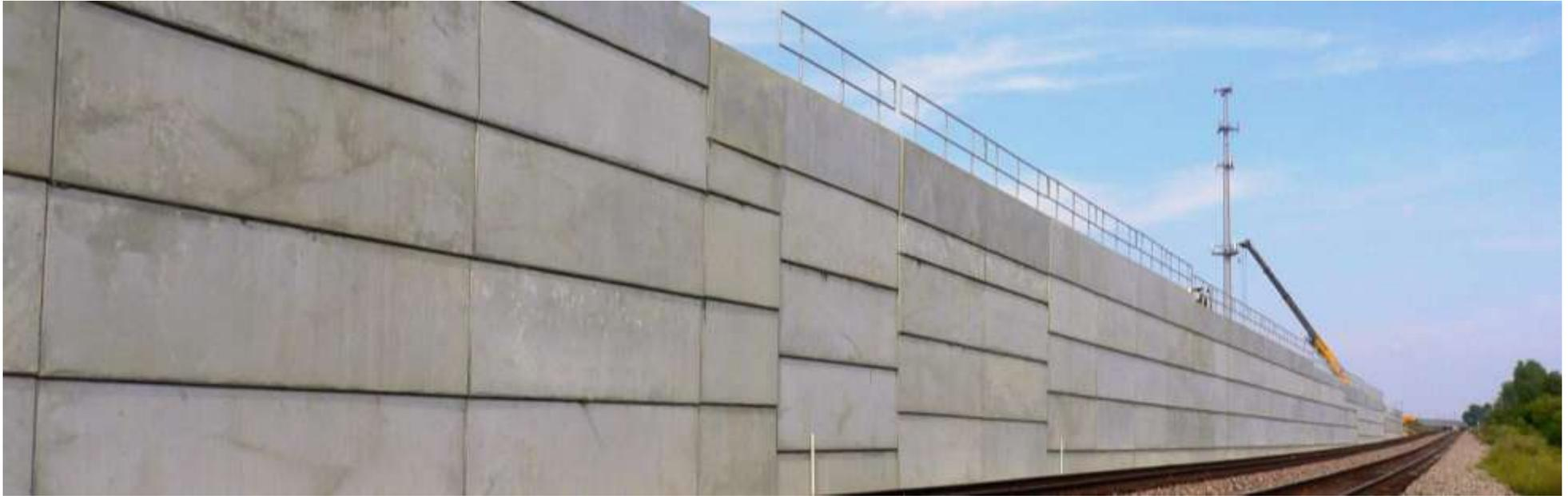
Typical EVERGREEN MAXI WALL in Olathe, Kansas: Grade separation for eliminating five level crossings.
